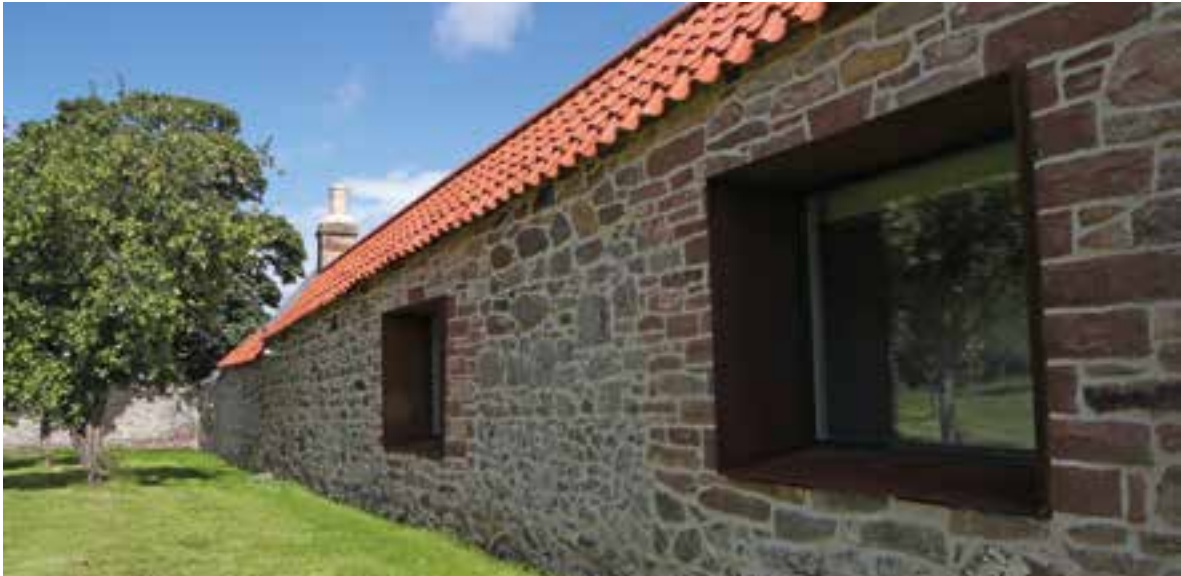
[Left] The owners didn't want to disguise the fact that these were once fully operational agricultural buildings, but some of the rougher edges have gone. Now it is the beauty of the stone that comes to the fore, with hints of the farm setting. The touches of green in this bedroom in the Byre, for instance, echo the expanse of fields and farmland beyond the windows
